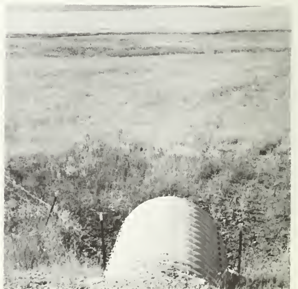
Looking West from WEST ENTRANCE
